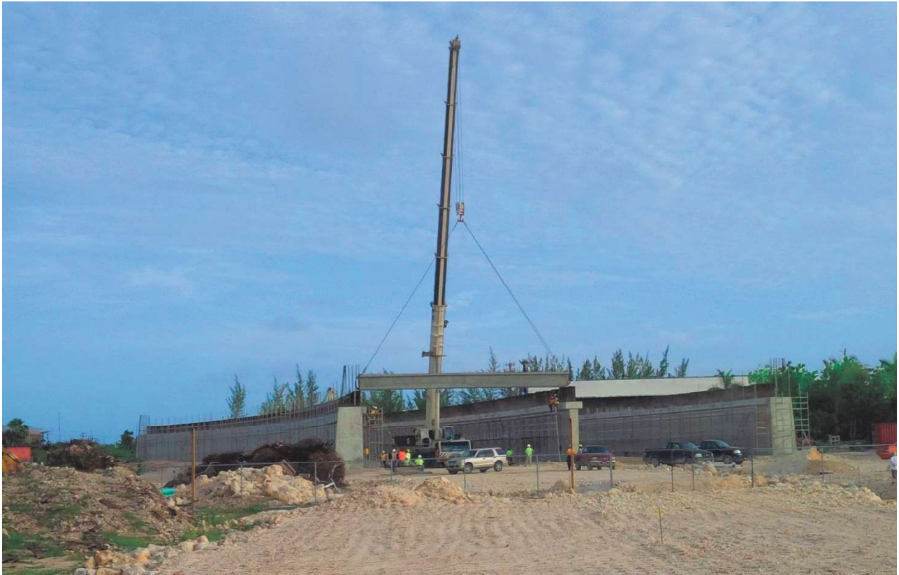
Figure 5: First bridge beam being installed at the ETH underpass
